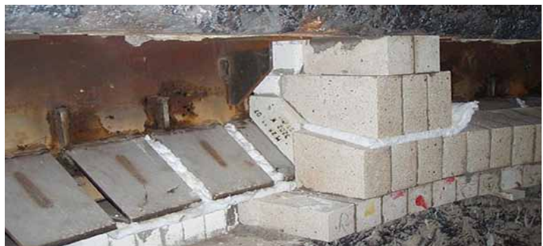
Above: Replacement of shaped console bricks in a round post combustion chamber.
