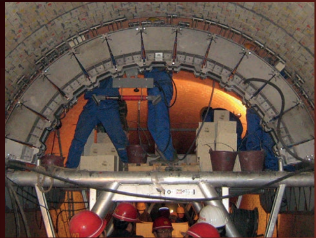
Above: Installation of STEULER-KCH refractory lining
