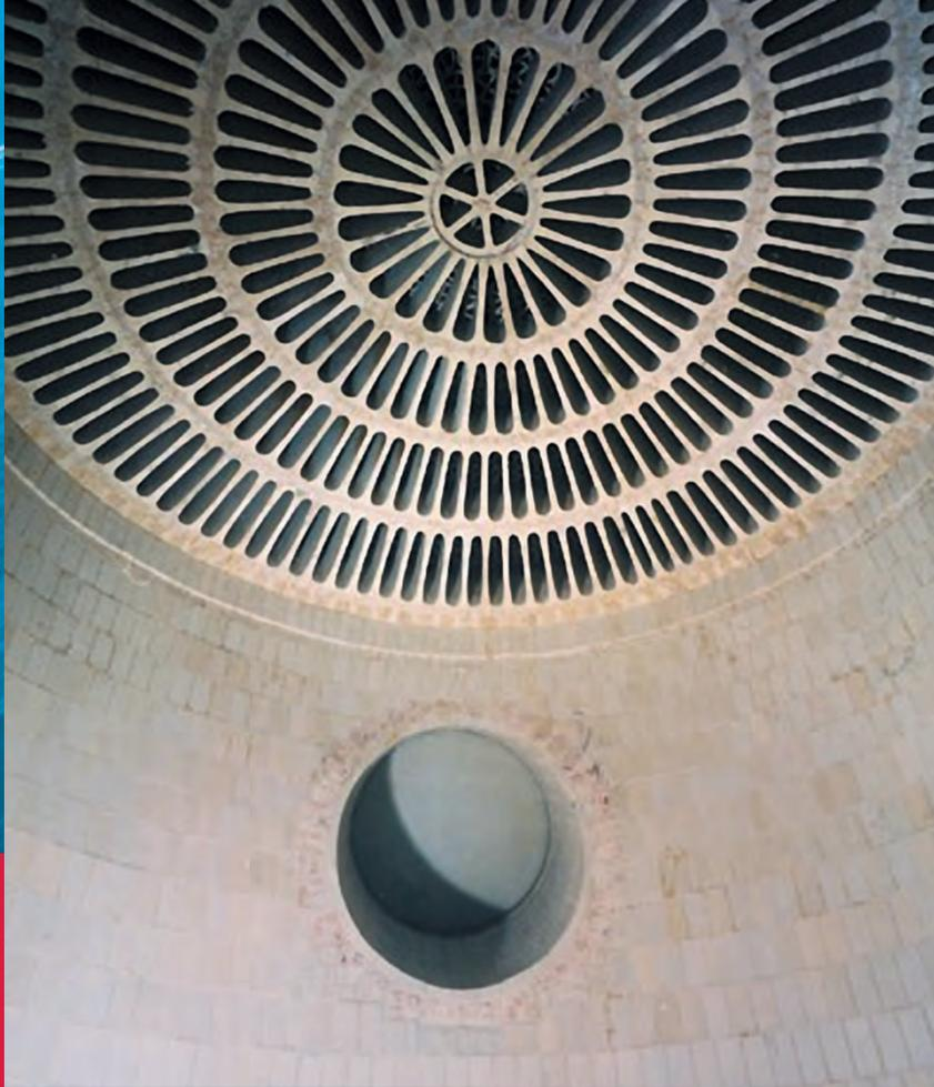
**Above:** Self supporting Steuler Dome constructed of acid proof ceramic, above a gas inlet.
