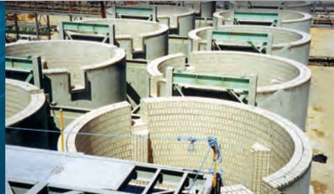
**Above:** Reactors lined with chemical and abrasion resistant linings.
