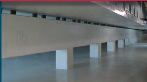
**Above:** Supporting concrete structures and floor surfaces beneath electrolysis cells are reliably protected with polyurethane coatings.
