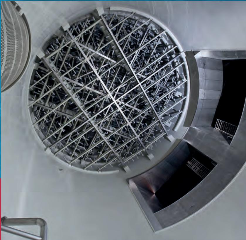
**Above:** Nozzle arrays and linings made of polypropylene in concrete flue gas scrubbers. Here one of two flue gas desulphurisation scrubbers for the 2,200 MW RWE lignite-fired power plants Neurath BoA II/III, built for AE&E.
