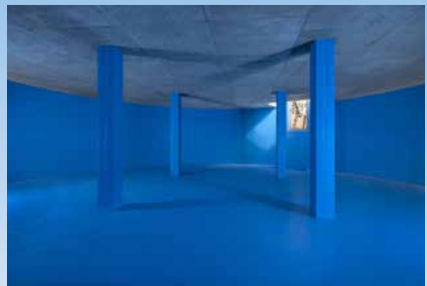
Above: Aqua-Lining 400 enables the completely lined potable water tank to meet hygiene requirements while reducing maintenance costs and extending service life.
