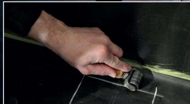
Application of a rubber lining.
