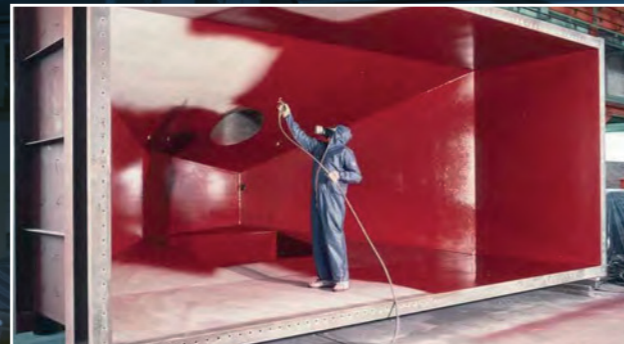
Spray application of a coating with barrier fillers.
