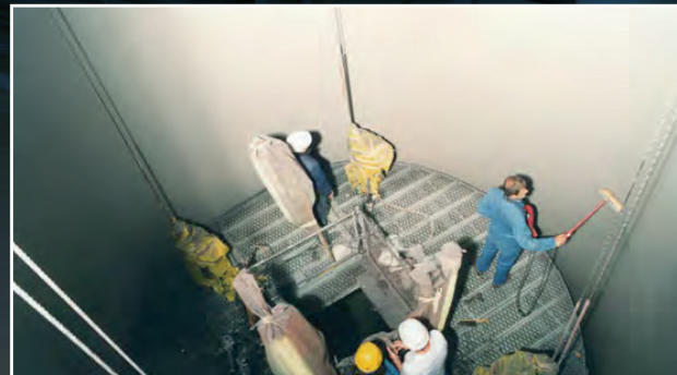
Leak testing of a chimney coating.
