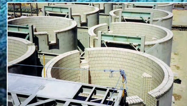
System lining with ceramic bricks.
