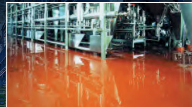
Floor coating in a chemical plant.
