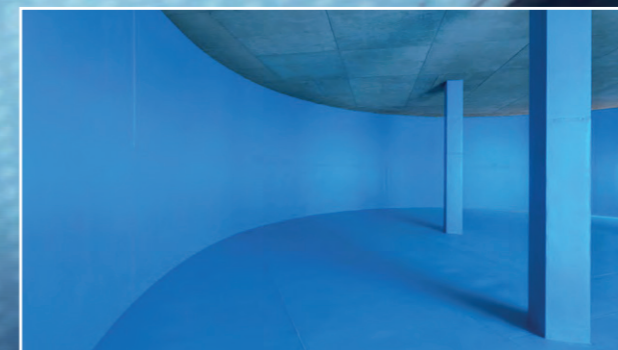
BEKAPLAST AQUA LINING in a drinking water reservoir.
