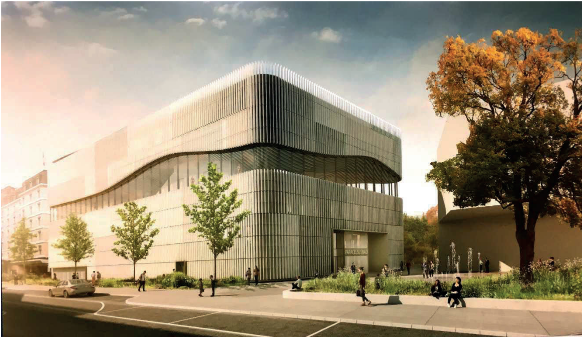
The view from the sports pool of the Paracelsusbad offers fascinating vistas of the Salzburg Fortress Illustration: BERGER+ PARKKINEN Architects
